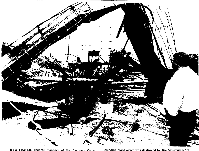
REX FISHER, general manager of the Farmers Co-op Elevator, looks over the smoldering remains of a fertilizer blending plant which was destroyed by fire Saturday night in Allen. A leg tower was toppled by the heat from the fire.
